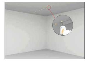
Prepare 10 mm thick wooden blocks. thickness, with a size that matches that matches the interior space of the tubes of wood. Fix the wooden blocks on the top of the installation site to an appropriate interval.
